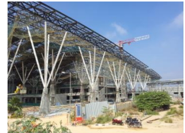
Expansion work in progress
