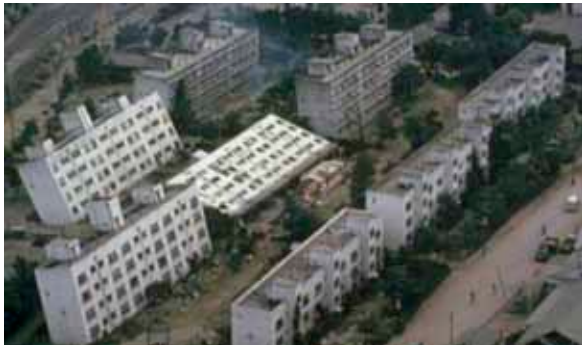
Fig. 6 :Toppling of Apartment buildings at Kawagishi Cho due to foundation soil liquefaction during Niigata earthquake of 1964
