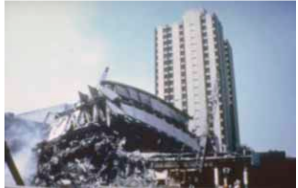
Fig. 7: Total collapse of 21-story steel frame office Building and building standing in background during Mexico earthquake of 1985
