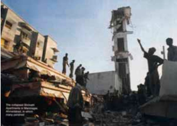
Fig. 13: Lift portion of an apartment building intact while the rest of the structure has collapsed in Ahmedabad during Bhuj earthquake of 2001
