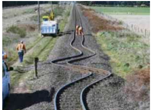
Fig. 8: Railway track subjected to shear due to ground movement during Canterbury earthquake of 2010
