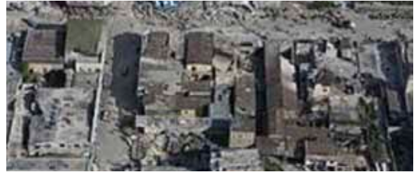
Fig. 4: Down town area of Port Au Prince, capital city of Haiti after the earthquake in 2010
