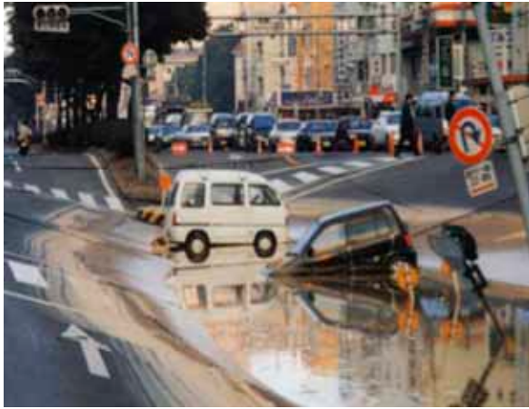
Fig. 5: Effect of liquefaction and collapse of underground metro station during Kobe earthquake of 1995
