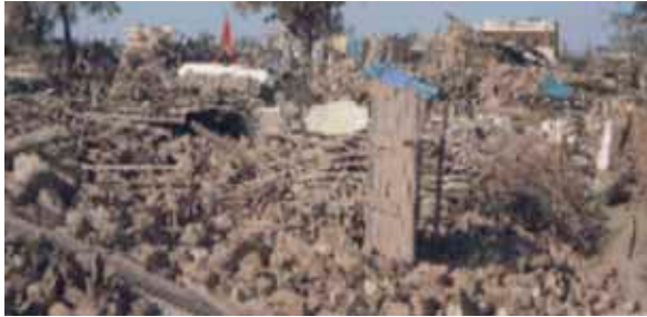
Fig. 3: Rapar town in Gujarat reduced to rubble after the Bhuj earthquake of 2001
